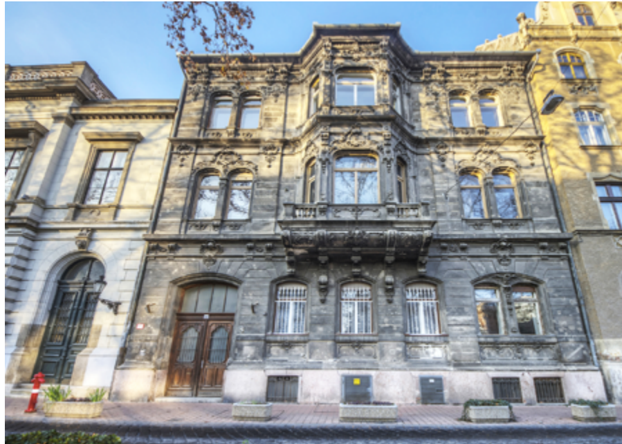
Brody House aussen
